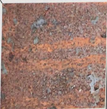
RUSTY STEEL ACCENT BEAMS
